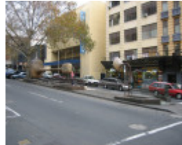
H2108 Underground Toilets Melbourne 08 06 06 mz 050
