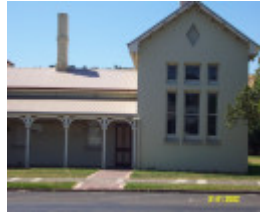
23063 Wannon Shire Offices Coleraine 0428
