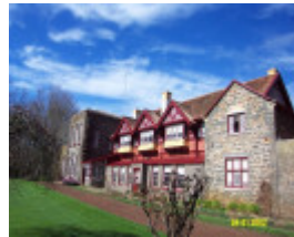
H0289 Murndal facade from NW 1318
