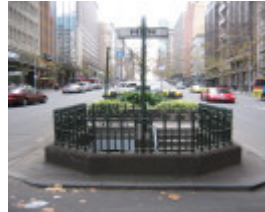
H2109 Underground Toilet Queen St 08 06 06 mz 018
