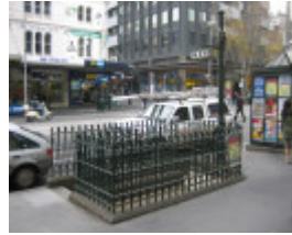
Underground men's toilet Elizabeth St GPO 08 06 06 mz 028
