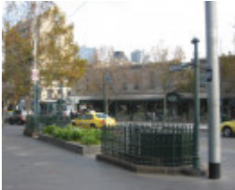
H2111 Underground Toilets Elizabeth & Victoria Sts 08 06 06 mz 004
