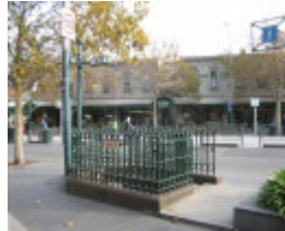
H2111 Underground Toilets Elizabeth & Victoria Sts 08 06 06 mz 001
