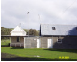
23094 Showgrounds Coleraine Office and Hall 1263
