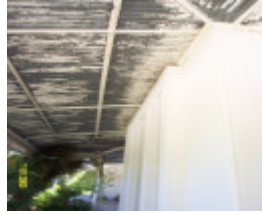
H0361 Kongbool verandah roof 2379
