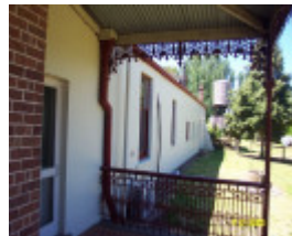
23123 Englefield Balmoral north verandah 2305
