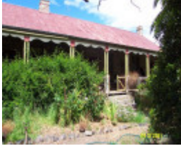
23132 Clunie Homestead front verandah 0270
