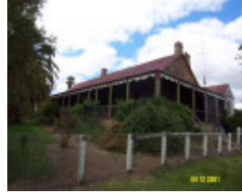
23132 Clunie Homestead front verandah 0271
