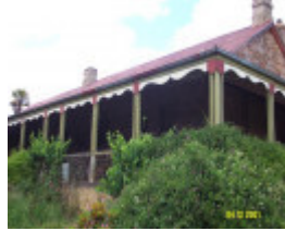
23132 Clunie Homestead front verandah 0272
