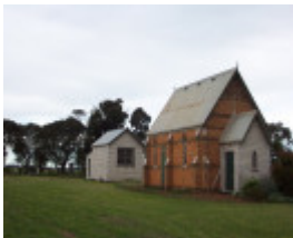
23140 Zion Lutheran Church Byaduk 0077
