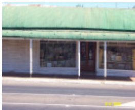
23144 store curved roof 0412
