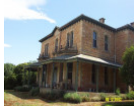
H1925 Gringegalgonia Homestead facade 2208
