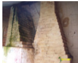
23162 Spring Vale Kitchen chimneys 0237
