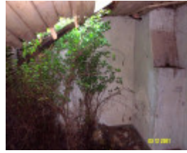
23162 Springvale Coojar timber section 0222
