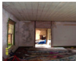
23162 Springvale Coojar brick section 0217
