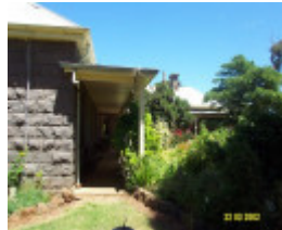
23187 Warrayure Homestead Complex rear 1885
