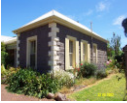
23187 Warrayure Homestead Complex side windows 1882
