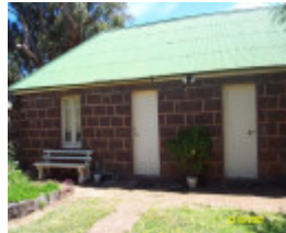
23187 Warrayure Homestead Complex gaol 1892
