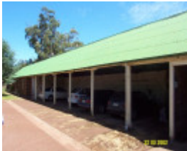
23187 Warrayure Homestead Complex machinery shed 1889
