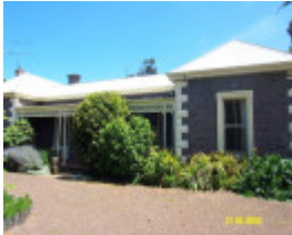
23187 Warrayure Homestead Complex facade 1878
