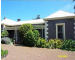
23187 Warrayure Homestead Complex facade 1878
