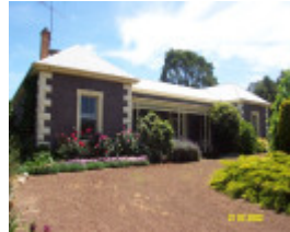
23187 Warrayure Homestead Complex facade 1879
