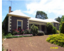
23187 Warrayure Homestead Complex facade 1879
