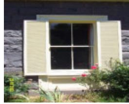
23187 Warrayure Homestead Complex window 1884
