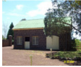
23187 Warrayure Homestead Complex stables 1886
