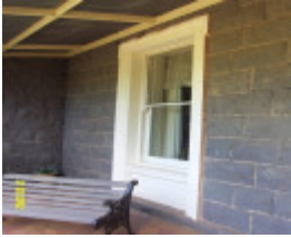
23187 Warrayure Homestead Complex window 1876
