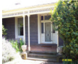
23187 Warrayure Homestead Complex front door 1877
