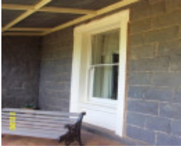
23187 Warrayure Homestead Complex window 1876
