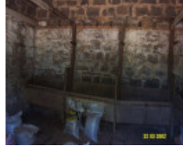
23187 Warrayure Homestead Complex stable 1887
