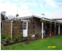
23190 Lyne Homestead Byaduk North side elevation 1435
