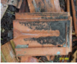
23192 Bassett Homestead Branxholme roof tile 1412
