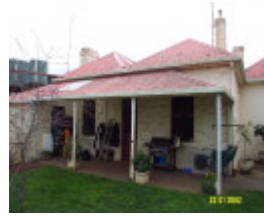
23192 Bassett Homestead Branxholme side elevation 1420
