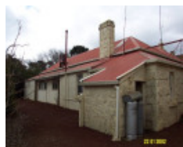
23192 Bassett Homestead Branxholme rear elevation 1418
