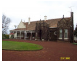
23192 Bassett Homestead Branxholme front elevation 1407
