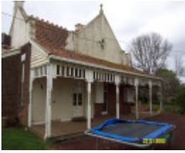
23192 Bassett Homestead Branxholme side elevation 1403
