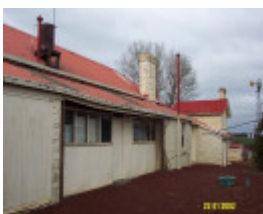
23192 Bassett Homestead Branxholme rear elevation 1417
