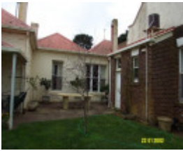
23192 Bassett Homestead Branxholme side elevation 1421
