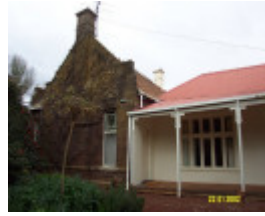
23192 Bassett Homestead Branxholme side elevation 1413
