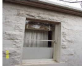
23192 Bassett Homestead Branxholme side elevation 1415
