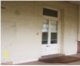
23192 Bassett Homestead Branxholme side elevation 1404
