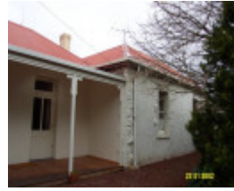
23192 Bassett Homestead Branxholme side elevation 1414
