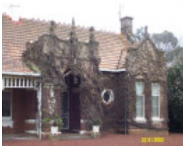
23192 Bassett Homestead Branxholme front elevation 1406
