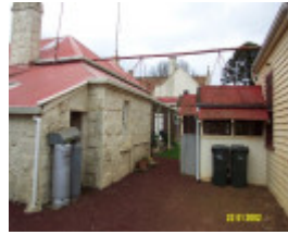
23192 Bassett Homestead Branxholme side elevation 1419
