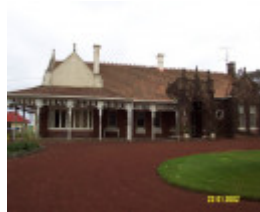
23192 Bassett Homestead Branxholme front elevation 1405
