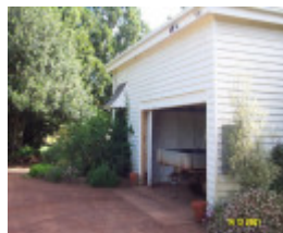
23196 Clifton Homestead rooms converted to garage 0324
