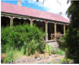
23196 Clunie Homestead front verandah 0270
