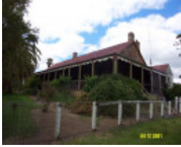
23196 Clunie Homestead front verandah 0271
