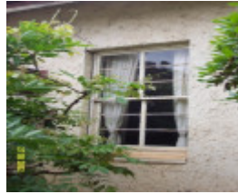
23205 Springwood Homestead Wannan window detail 2057
