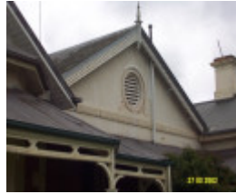
23205 Springwood Homestead Wannan gable detail 2051
