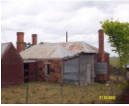
23205 Springwood Homestead Wannan stone cottage 2063
