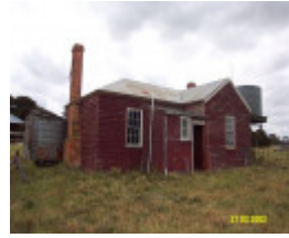
23205 Springwood Homestead Wannan stone cottage extension 2070
