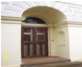
23205 Springwood Homestead Wannan entrance 2049
