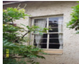
23205 Springwood Homestead Wannan window detail 2057
