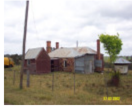
23205 Springwood Homestead Wannan stone cottage 2064
