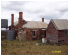
23205 Springwood Homestead Wannan stone cottage rear 2065
