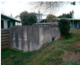
h01090 fort franklin portsea bunker 01 0903 mz
