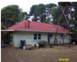
23230 Dunroe Byaduk North garage rear 0051
