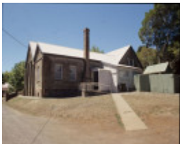
Christ Church School_Daylesford_South Elevation_Feb 2004_mz
