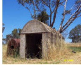
23254 Timber Kiln and Boiler Balmoral 2096
