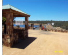
23255 Rocklands Reservoir dam wall 2084
