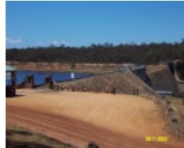
23255 Rocklands Reservoir dam wall 2083
