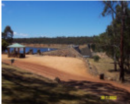
23255 Rocklands Reservoir dam wall 2082
