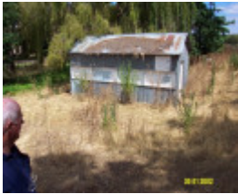
23286 Swimming Pool Byaduk kiosk 0386
