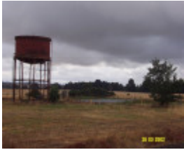
23291 Railway Water tower Branxholme 0559
