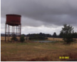
23291 Railway Water tower Branxholme 0559
