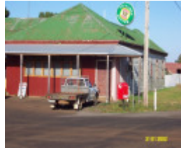
23295 Junction Hotel Branxholme 0470
