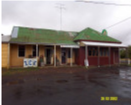
23295 Junction Hotel Branxholme 0563
