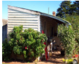
23304 Brae Park Branxholme shed 0722
