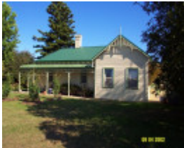
23304 Brae Park Branxholme north side 0724
