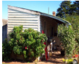
23304 Brae Park Branxholme shed 0722
