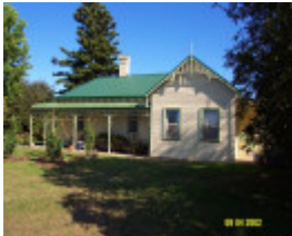
23304 Brae Park Branxholme north side 0724
