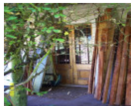
23310 Timber House Branxholme verandah 0719
