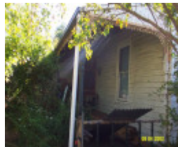
23310 Timber House Branxholme verandah 0718
