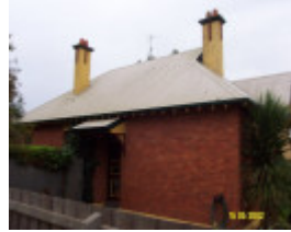
23332 Police Residence Martin St Penshurst S side 1005
