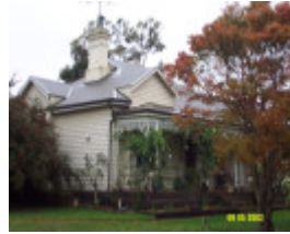
23360 School Master s Residence Former 59 Bell St Penshurst 0917
