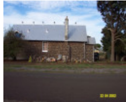
23363 State School 486 Former 67 Watton St Penshurst 0822
