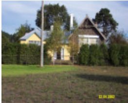
23363 State School 486 Former 67 Watton St Penshurst 0819
