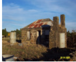
23373 Groves Cottage Watton street Penshurst 0891
