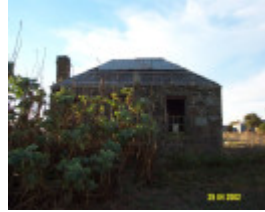
23373 Groves Cottage Watton street Penshurst 0889
