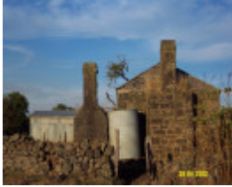
23373 Groves Cottage Watton street Penshurst 0890
