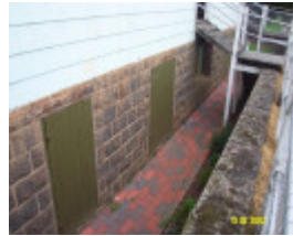
23379 Grandstand Racecourse Penshurst bar toilets 1543
