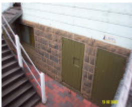
23379 Grandstand Racecourse Penshurst bar toilets 1544
