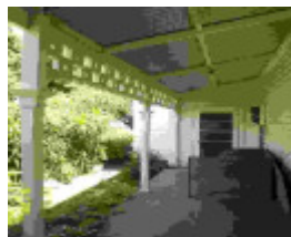
23400 Riverside Side verandah 0182
