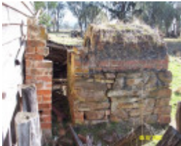
23404 Ruined House Mirranatwa oven 1139
