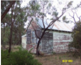
23416 Former School Mooralla 1176
