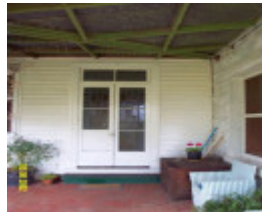
23419 Lovatdale Glenthompson detail of verandah 1234
