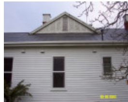
23419 Lovatdale Glenthompson west elevation 1238
