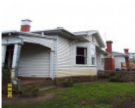
23419 Lovatdale Glenthompson west elevation 1229
