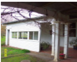
23419 Lovatdale Glenthompson detail of verandah 1235
