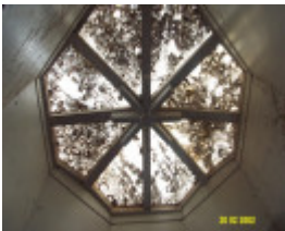
23435 Skene Homestead Strathkellar 1858 skylight 1613
