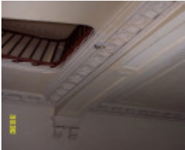
23435 Skene Homestead Strathkellar 1858 hall ceiling 1583
