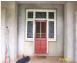
23435 Skene Homestead Strathkellar 1923 front door 1567
