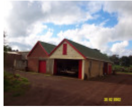
23435 Skene Homestead Strathkellar garages
