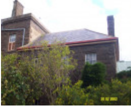
23435 Skene Homestead Strathkellar 1880s billiard room 1572
