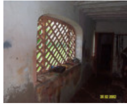
23435 Skene Homestead Strathkellar stables 1626
