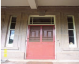
23435 Skene Homestead Strathkellar 1858 front door 1556
