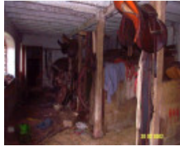
23435 Skene Homestead Strathkellar stables 1625
