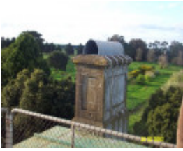
23435 Skene Homestead Strathkellar 1858 chimney 1612
