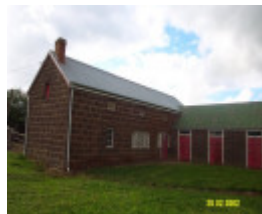
23435 Skene Homestead Strathkellar stables 1573
