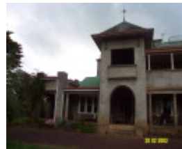
23435 Skene Homestead Strathkellar 1923 tower 1560
