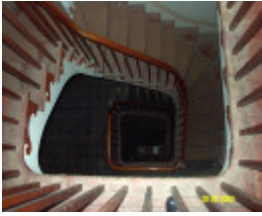
23435 Skene Homestead Strathkellar 1858 staircase 1615
