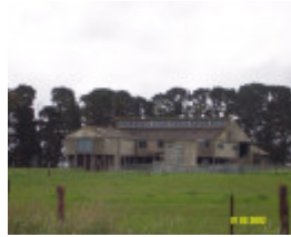
23441 Torbank Woolshed Tobermory Rd Penshurst 1715
