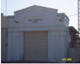
23449 Fire Station Coleraine 0462
