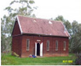
23450 CofE Former Scouts Hall Wannon 1338
