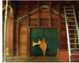
23450 CofE Former Scouts Hall Wannon 1340
