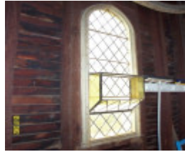
23450 CofE Former Scouts Hall Wannon 1341
