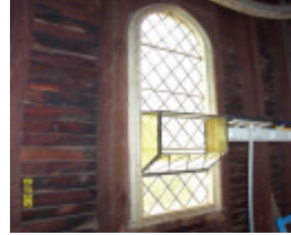
23450 CofE Former Scouts Hall Wannon 1341
