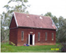
23450 CofE Former Scouts Hall Wannon 1338
