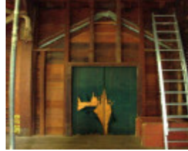
23450 CofE Former Scouts Hall Wannon 1340
