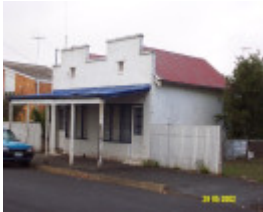
23454 Turner s Store Residence Glenthompson 1050
