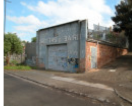
Maribrnong Battery Maribrnong May 2003 Griffith And Baird Engineers Toolshop
