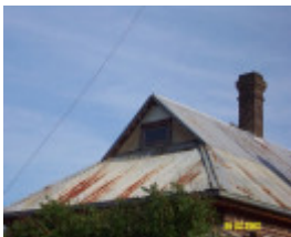
23480 Myrning Wootong Vale roof detail 2007
