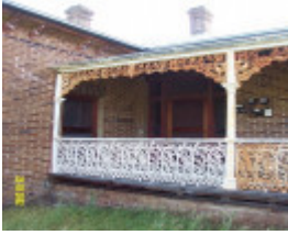
23480 Myrniong Wootong Vale verandah 1997
