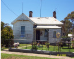
23481 Police station residence former Balmoral 2098
