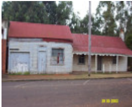
23483 Stewart s Store Residence Station St Glenthompson 1064
