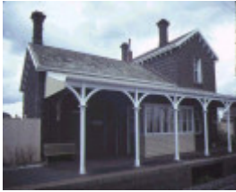
Source: Victorian Heritage Register. Taken 1984.
