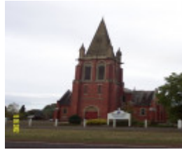
23498 St Michael s Lutheran Complex Tarrington church 0953
