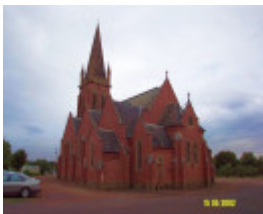
23498 St Michael s Lutheran Complex Tarrington church 0946
