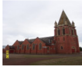
23498 St Michael s Lutheran Complex Tarrington church 0950
