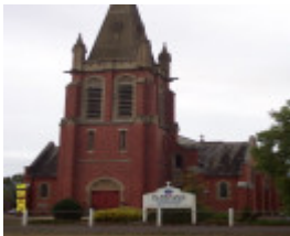
23498 St Michael s Lutheran Complex Tarrington church 0954
