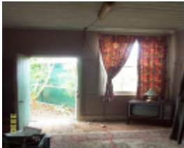
23499 Former School Gritjurk residence 2022
