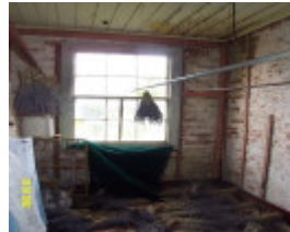
23499 Former School Gritjurk residence 2025
